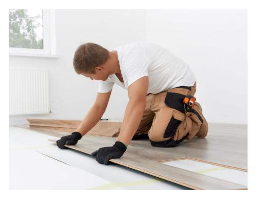
EcoDense® Flooring is a versatile flooring system that can be installed in most areas of your home. EcoDense® Flooring can be installed on, above or below grade levels.
